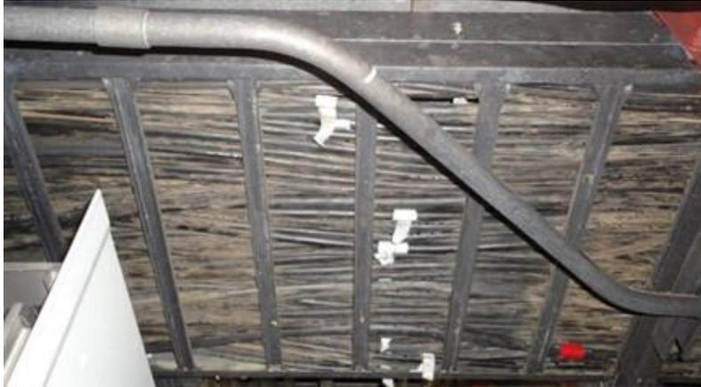
Harvesting field aged cables for additional temperature and radiation testing
