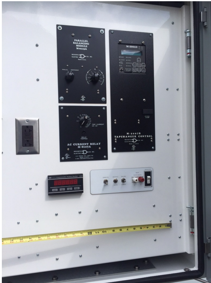
Figure 1 - LTC Controller with Traditional Circulating Current Equipment
