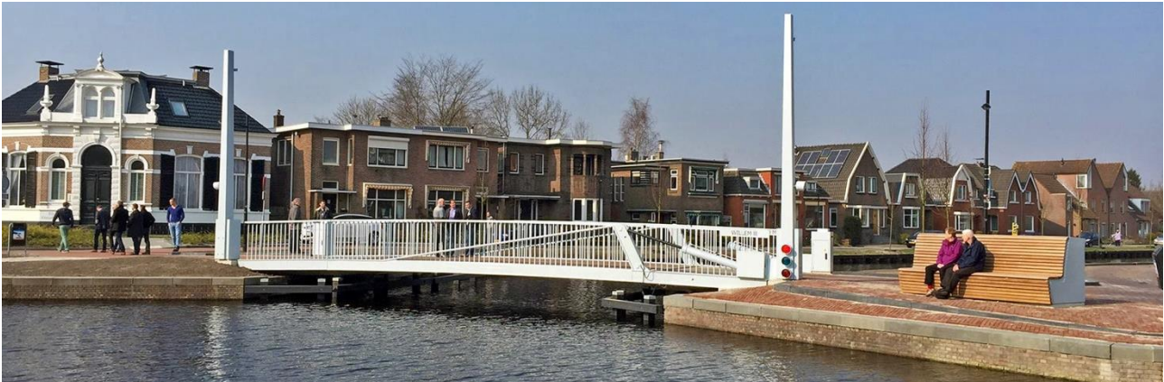
Fig. 13. Overview Willem III bridge Assen
