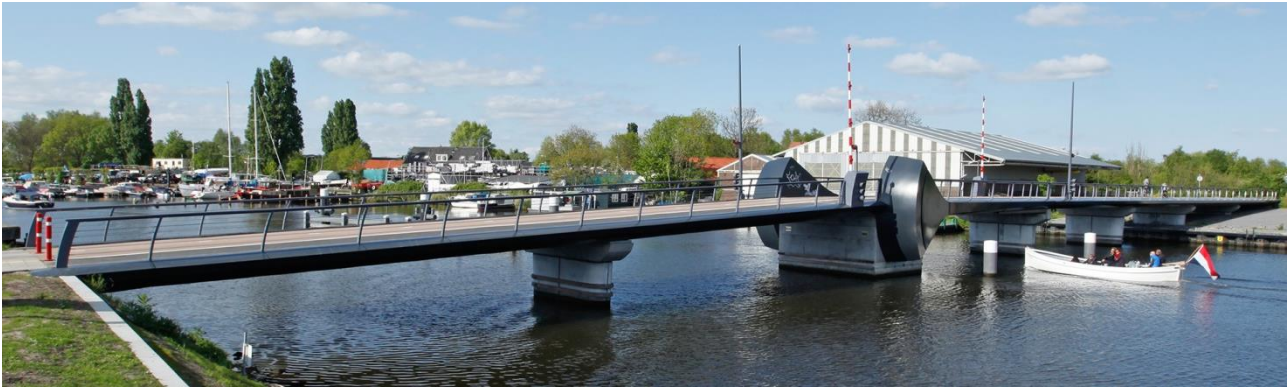
Fig. 9. Overview Kadoelen bridge Amsterdam
