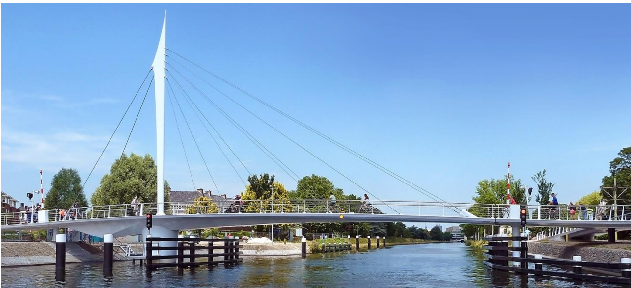
Fig. 1. Overview swing bridge Rijswijk
