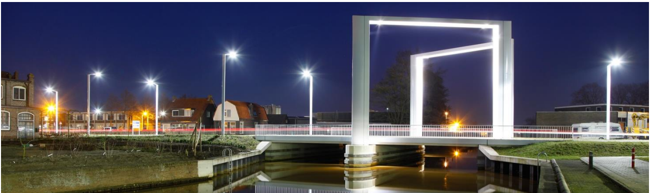
Fig. 14. Overview Dolder bridge Steenwijk
