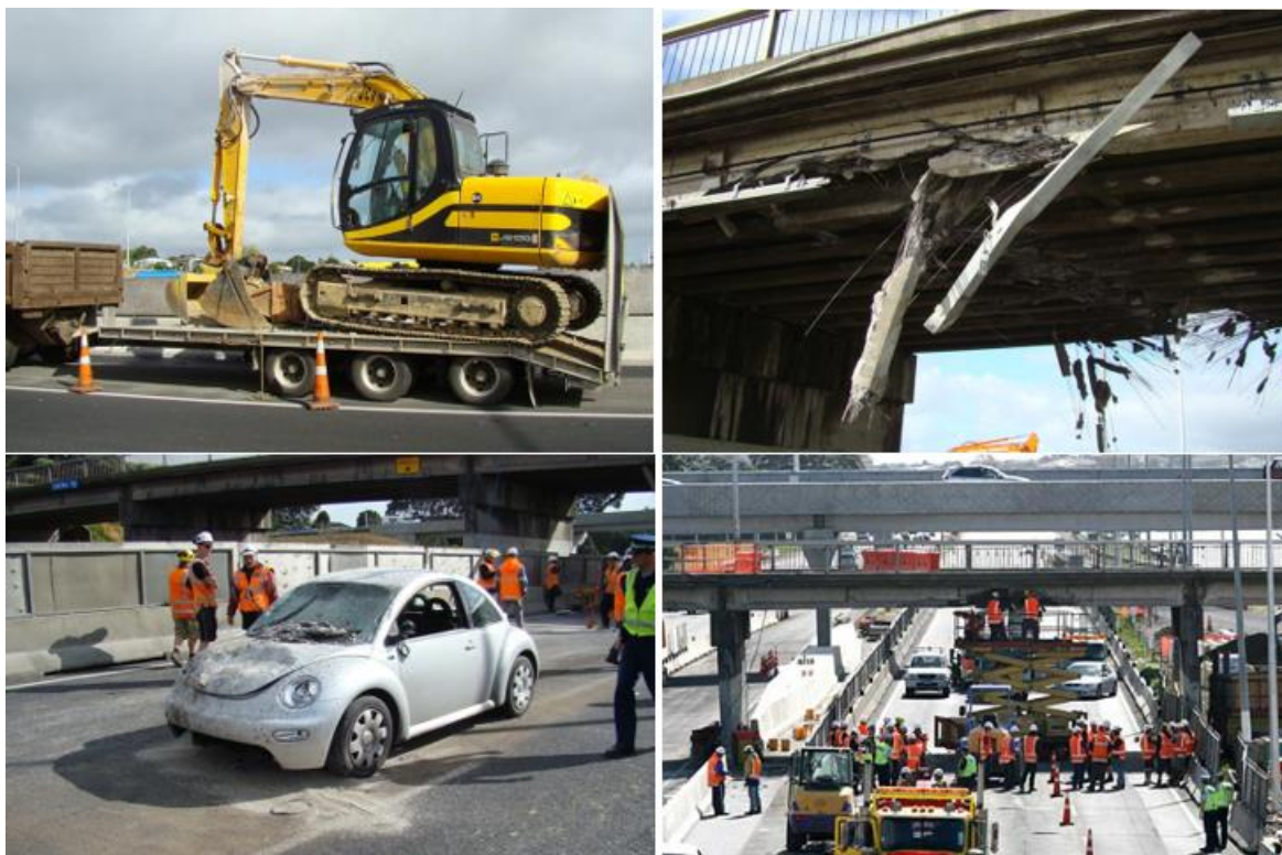
Figure 3 Onewa underpass 2009. (Source – Stuff.co.nz)
