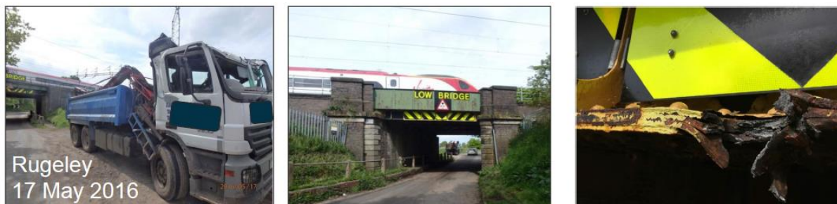
Figure 2 Photos of the Rugeley 2016 bridge strike. (Source - Network Rail)
