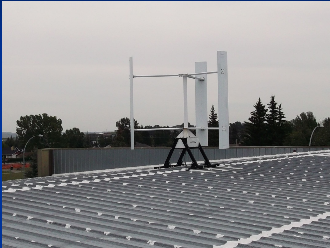
Vertical Axis Wind Turbine on the roof of the Oilfields Regional Arena
