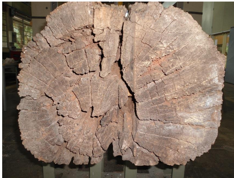
Figure 3 Radial drying cracks
