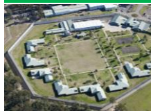
Outer Metropolitan Multipurpose Correctional Centre (OMMPCC), Sydney
