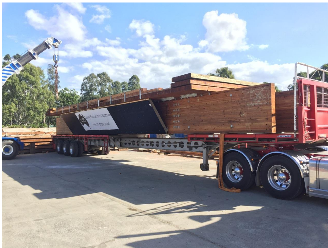
Figure 5 – Timber Restoration Systems glulam bridge pre-assembled for transport to a Queensland project
