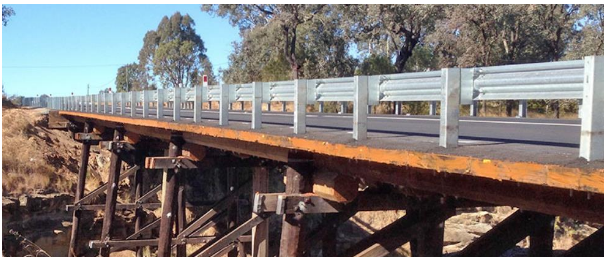
Figure 4 – PNG Forest Products NiuBridge system with plywood deck on the New England Highway
