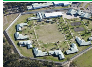
Outer Metropolitan Multipurpose Correctional Centre (OMMPCC), Sydney
