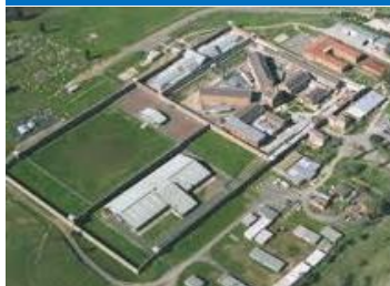
Goulburn Correctional Centre, Goulburn
