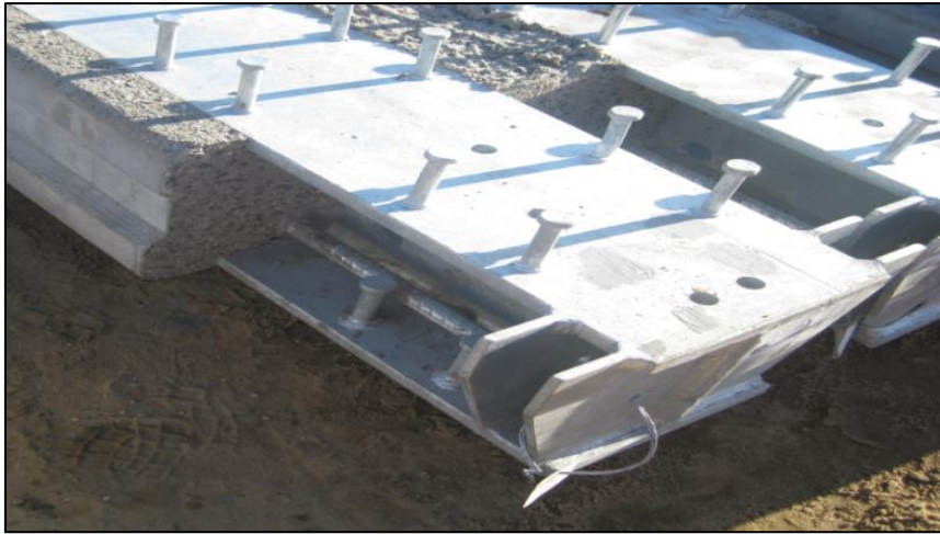
Figure 8 –Precast battledeck plank
