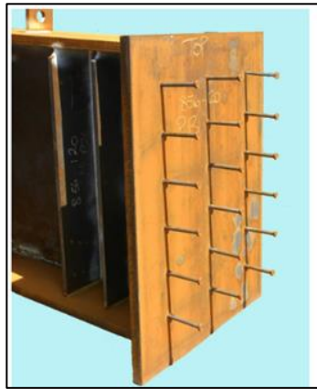
Figure 10 –End Plate Connection. [7]
