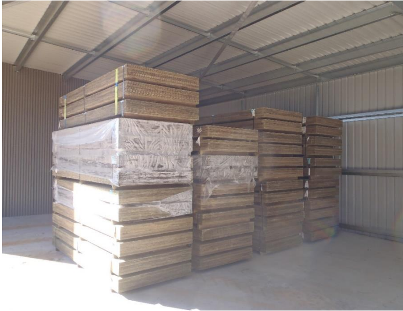
Bridgeply decking for Bailey bridging system
