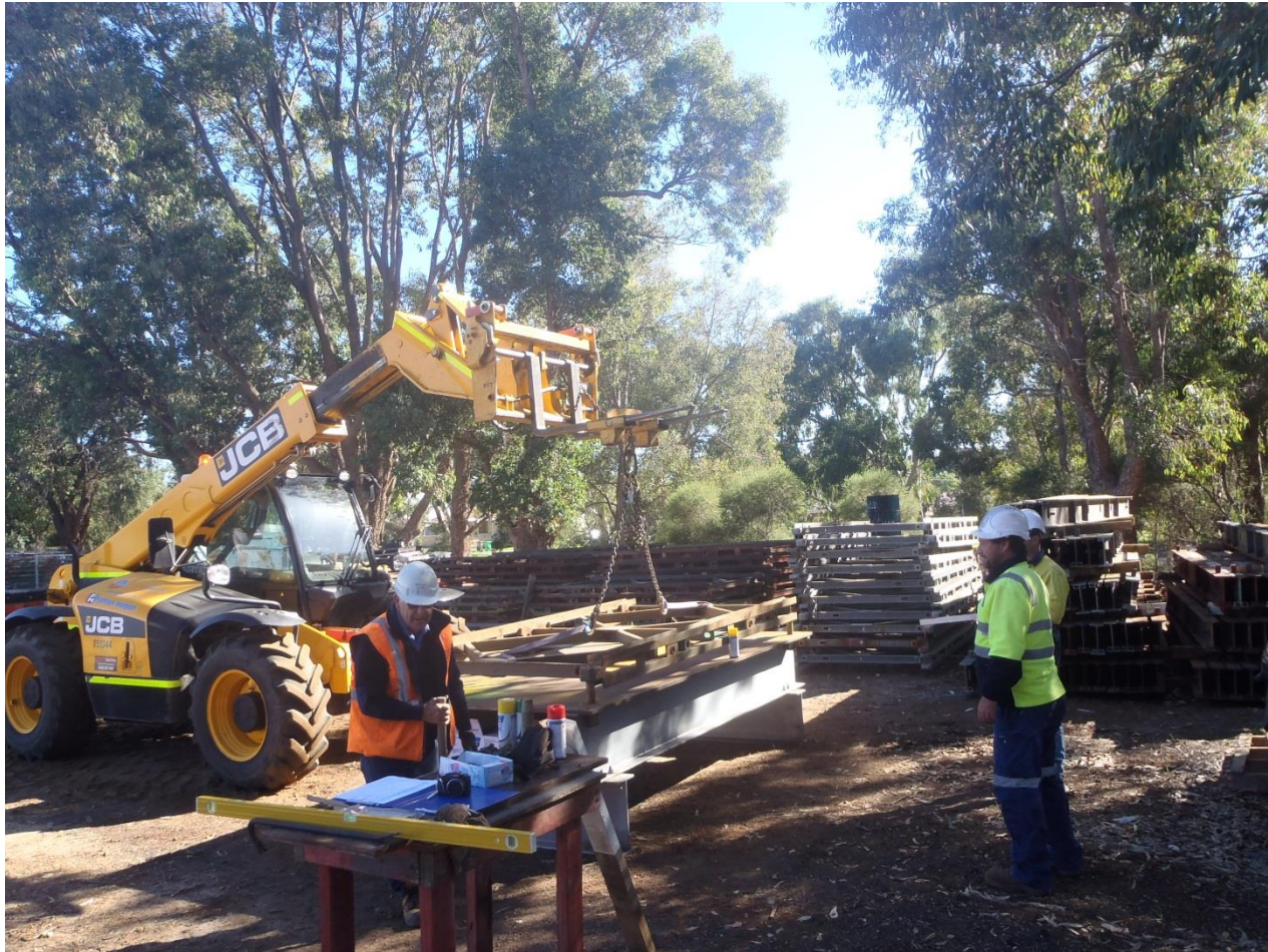
Placing panel on table
