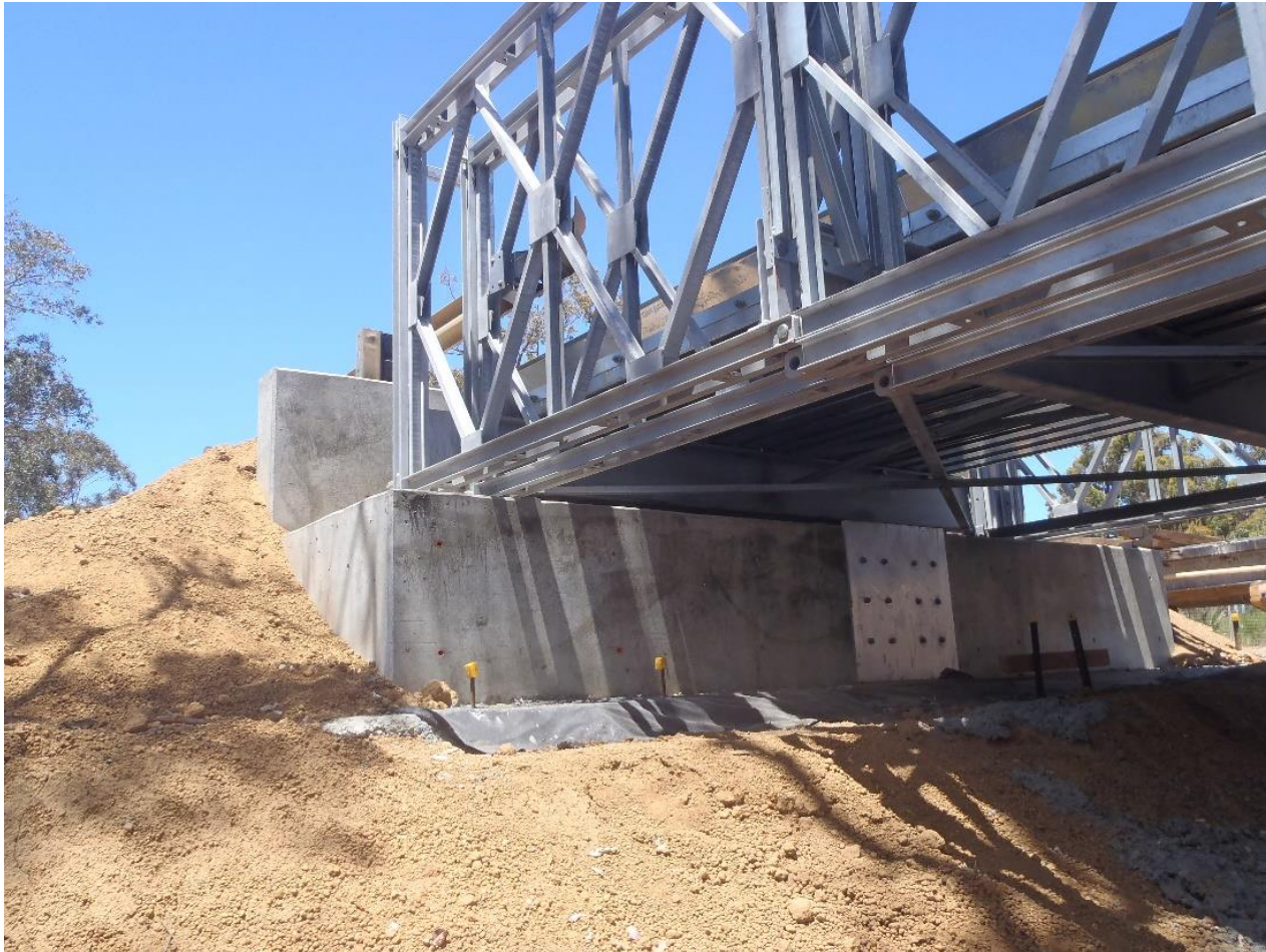
Precast Concrete Abutment for Mabey Compact 200
