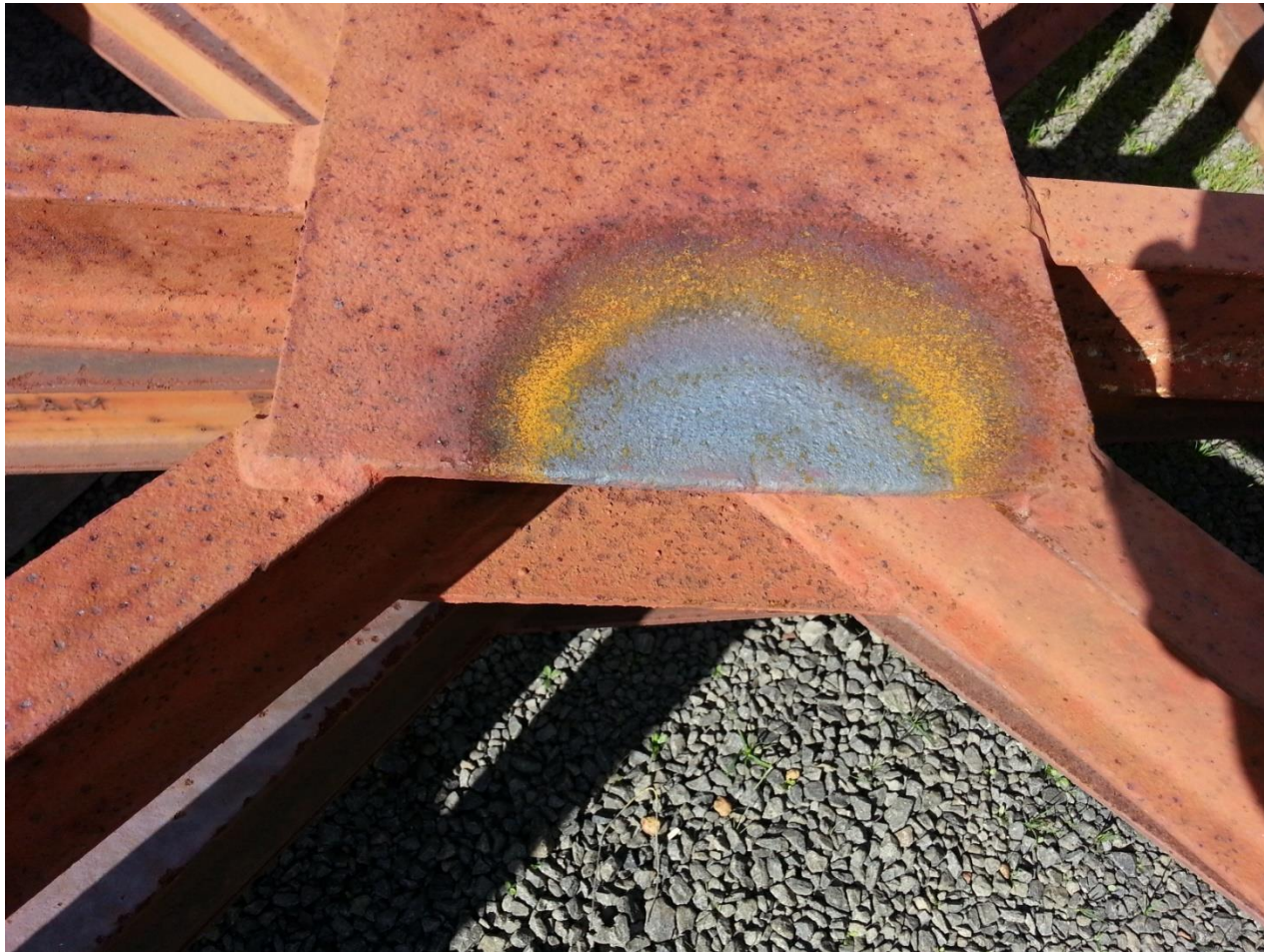
panel gusset plate straightened
