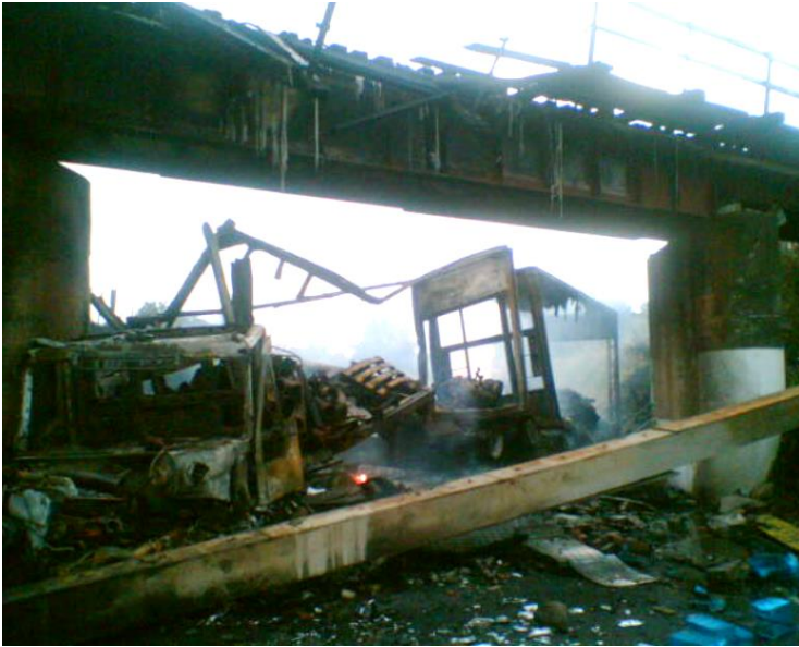
Picture 2 and 3 – A particularly bad example of damage to a span. The truck caught fire after it became wedged under a span of a rail bridge over SH1 near Marton. No-one was injured at this incident. (Photo Credit: Richard Greenfield)
