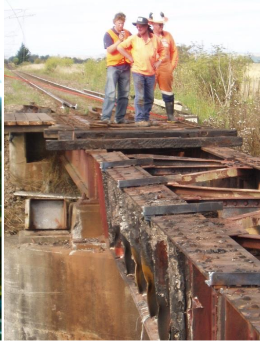
Picture 2 and 3 – A particularly bad example of damage to a span. The truck caught fire after it became wedged under a span of a rail bridge over SH1 near Marton. No-one was injured at this incident. (Photo Credit: Richard Greenfield)
