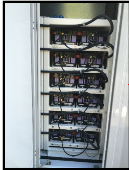
Battery Racks DC Switch
