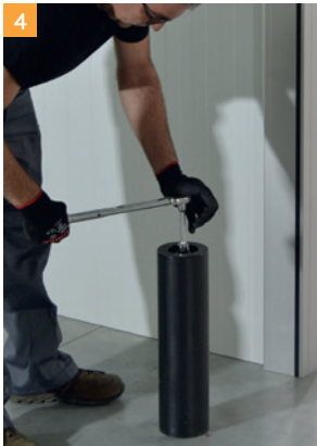
4 Locate anchor base and fix securely.
