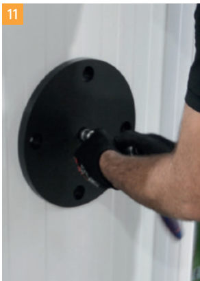
11 Securely fix reinforcement arm backing plate on other side of the wall.
