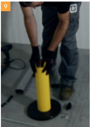
9 Assemble wall reinforcement arm components.
