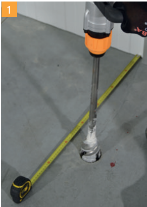
1 Measure and drill locations for anchor fixings.
